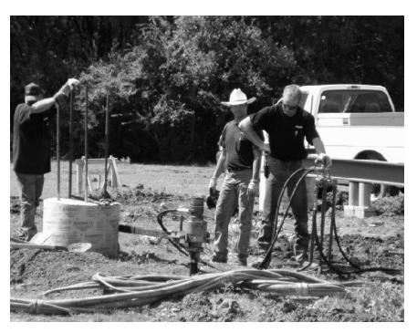
Figure 3.35- Installation of Helical Anchors
