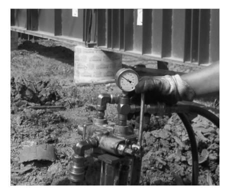
**Figure B4 - Measuring Pressure During Pressed Pile Installation**
