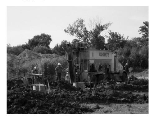
Figure 3.30- Pouring of Concrete Piers
