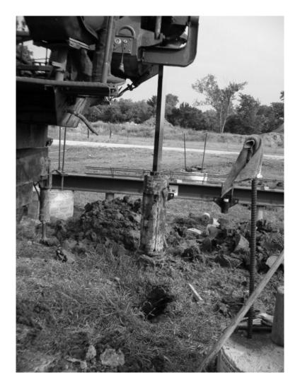
Figure 3.32- Installation of Belled Piers
