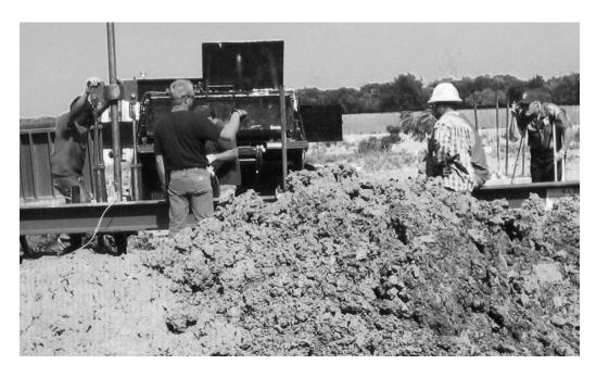
**Figure B3 - Installing Pressed Steel Piles**
