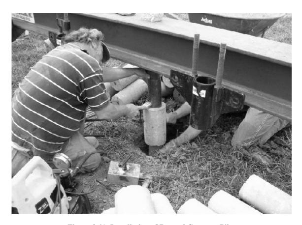
**Figure 3.41- Installation of Pressed Concrete Piles**
