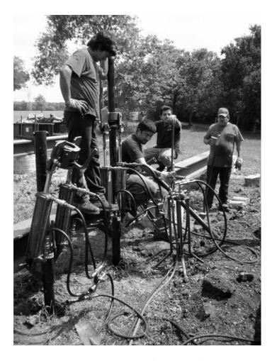
Figure 3.38- Installation of Pressed Steel Piles
