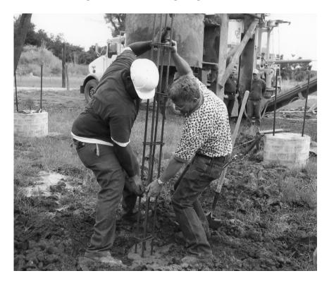
Figure B2 - Setting Steel For Augercast Piles
