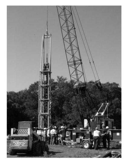
Figure 3.34- Installation of Augercast Piles
