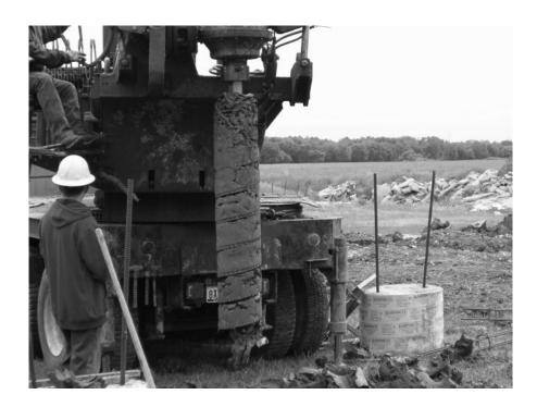
Figure 3.29- Drilled Shaft Installation
