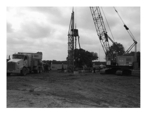
**Figure B1 - Installing Augercast Piles**
