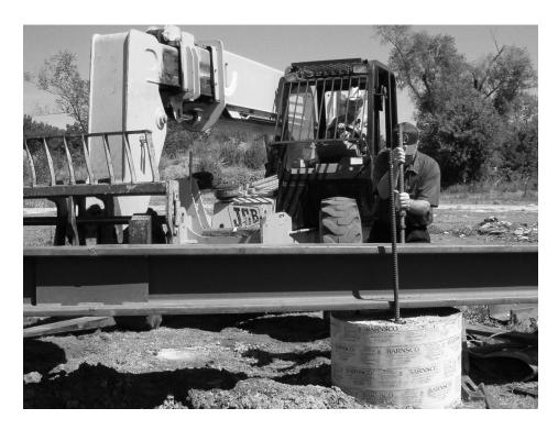
Figure 3.44 – Researcher Setting Coupled Tie-down Bar with Loader in Background
