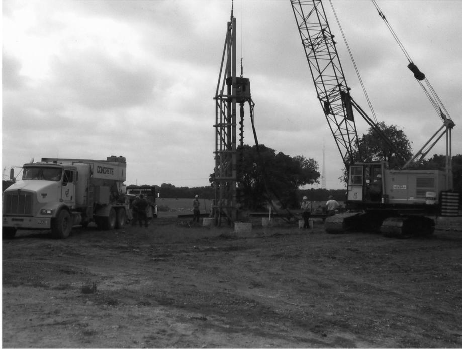
**Figure B1 - Installing Augercast Piles**
