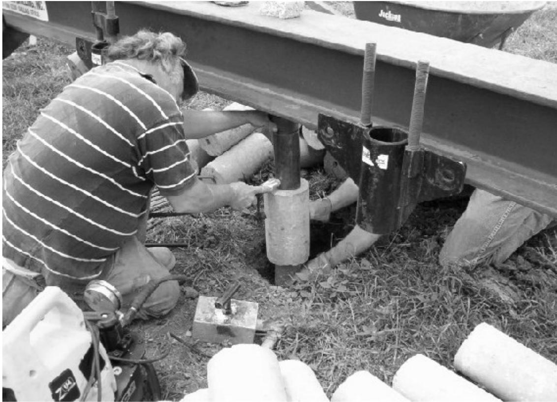
**Figure 3.41- Installation of Pressed Concrete Piles**
