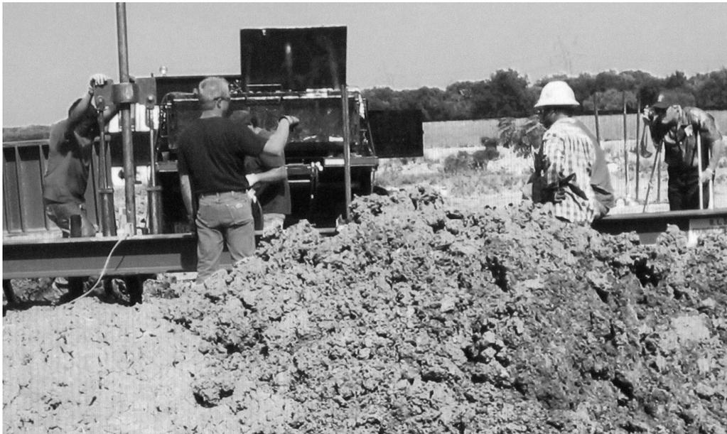
**Figure B3 - Installing Pressed Steel Piles**
