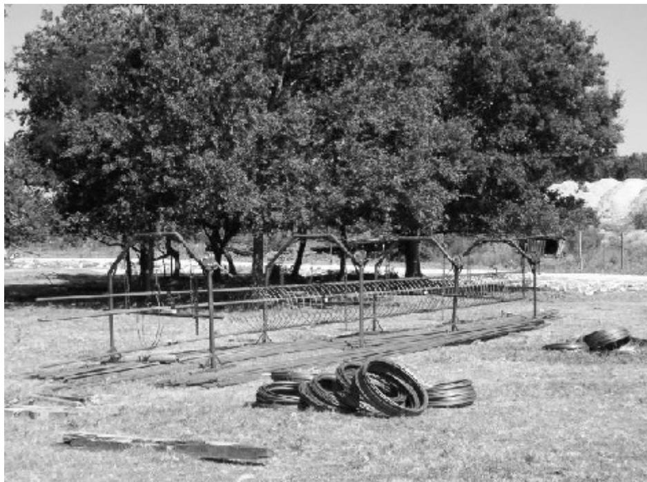
**Figure 3.23- Reinforcement Cages Being Tied for Reaction Piers**
