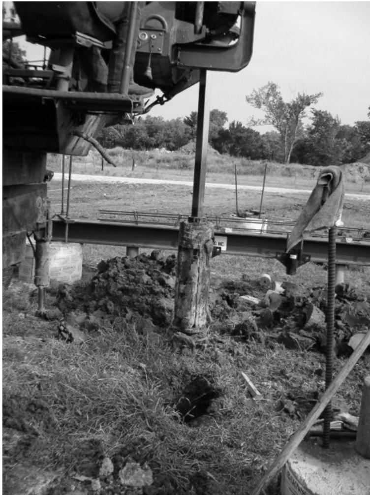
**Figure 3.32- Installation of Belled Piers**
