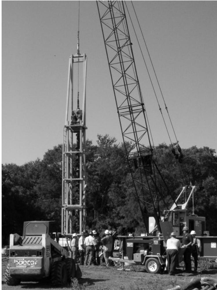
**Figure 3.34- Installation of Augercast Piles**
