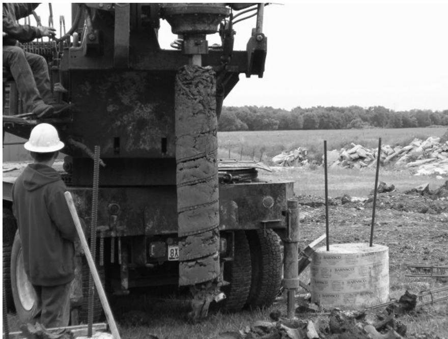
**Figure 3.29- Drilled Shaft Installation**
