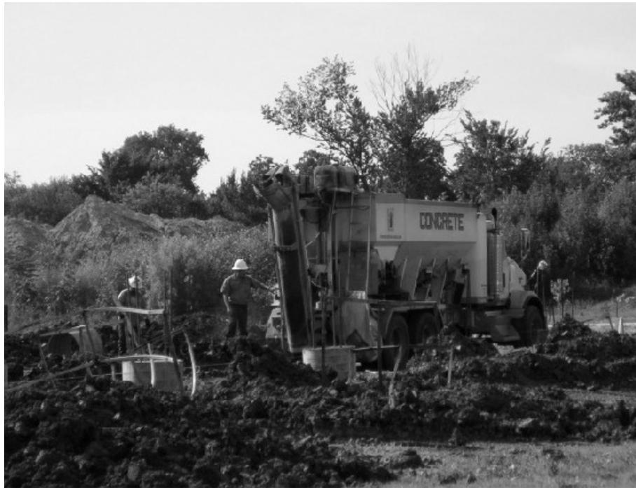
**Figure 3.30- Pouring of Concrete Piers**
