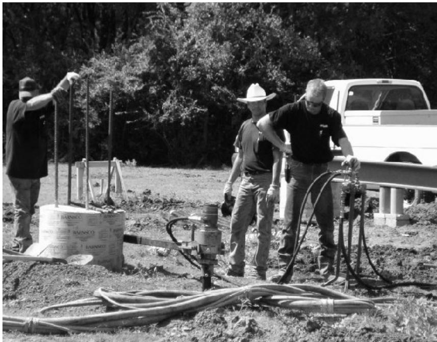
**Figure 3.35- Installation of Helical Anchors**
