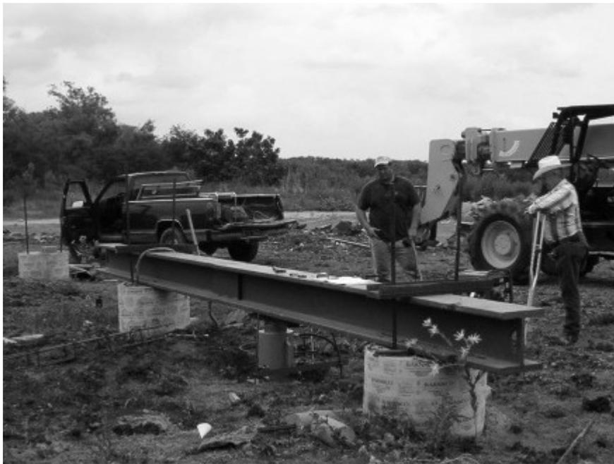
**Figure 4.4 – Load Testing of Belled Shafts**
