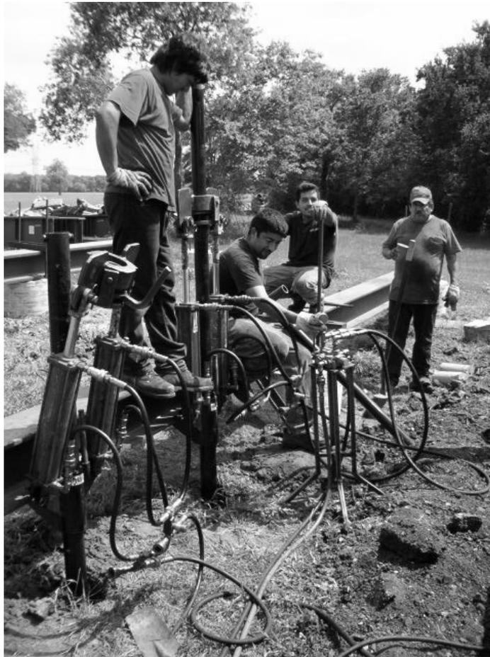
**Figure 3.38- Installation of Pressed Steel Piles**
